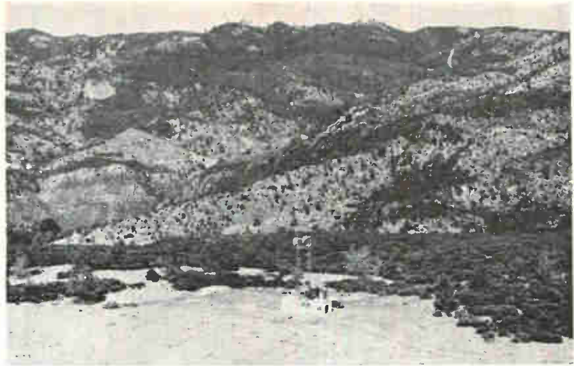
Western mountains dwarf microwave relay station as one more site is added to the more than 250 that will extend across the continent by 1962
