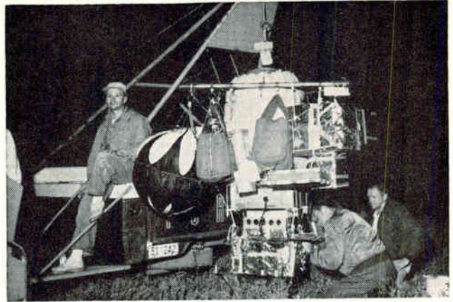
Balloon-borne cosmic-radiation telemetry gear of USAF's Aeromedical Field Lab is checked prior to launch.
