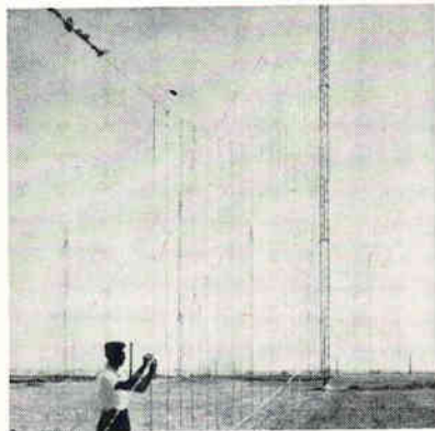
G/A Model 726 vertically polarized monopole log periodic antenna. VSWR of 2.1:1 (nominal). 10 db gain. Extremely low take-off angle. Several antennas can be arrayed to compress azimuth beamwidth.
