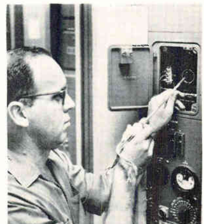
Traveling-wave tube for Bell System's satellite relay station amplifies signals as much as 10,000 times
