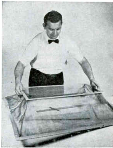
Mesh cloth is sewed into shield that covers a varying gap
