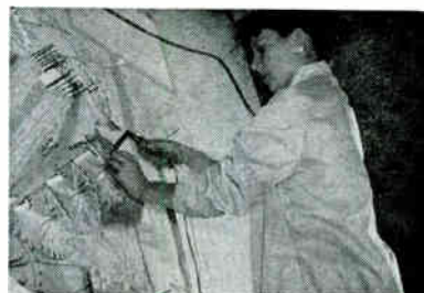
Women solderers also work on scaffold
