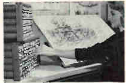
Harness wire dispensers are stacks of tubes
