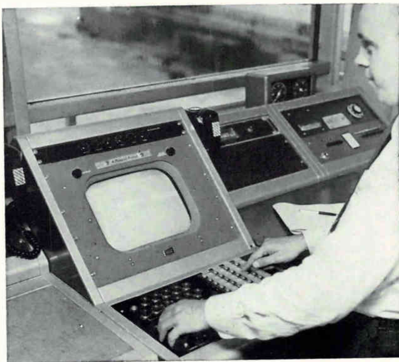
In Eastern Air Lines' big new passenger terminal at New York International Airport (Idlewild), all plane and vehicle movements on the apron, and all passenger information, are controlled from a coordinator's tower. Dage tv system keeps coordinator in touch with remote flight-information boards; keyboard lets him enter data on boards. Radio, Telautograph and other communication systems complete tower facilities
