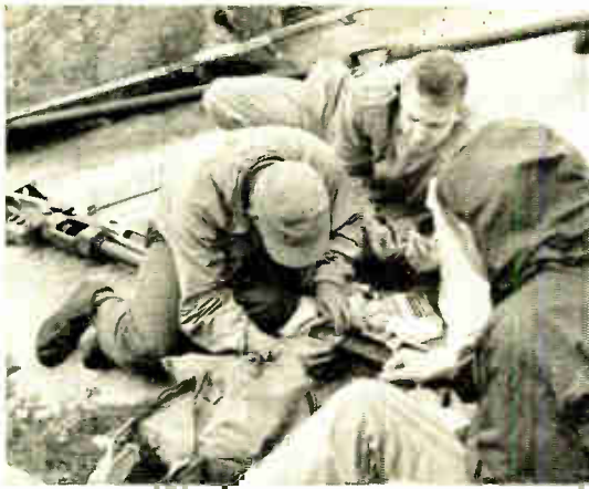
Engineers prepare reinforcing rod for strain gage installation atop The Old Man of the Mountains in New Hampshire
