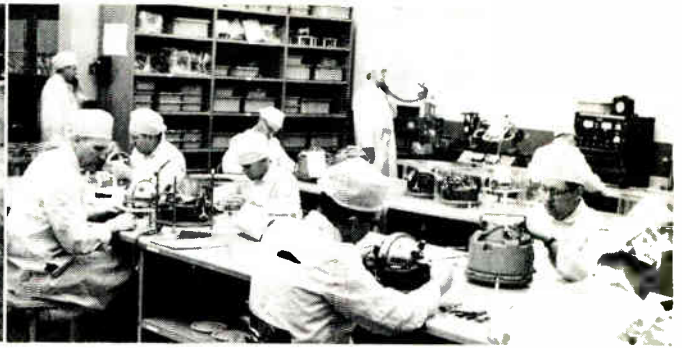
COMPLETE FACILITIES include dust-free rooms for precision production . . . environmental testing equipment . . . compass-testing devices that simulate ship's pitch, yaw and roll. Plant is fully air-conditioned.
