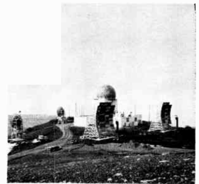
One of six new DEWline radar stations just completed by USAF along the Aleutian Island chain. Purpose is to prevent Soviet bombers from making an undetected end run around the northern DEWline
