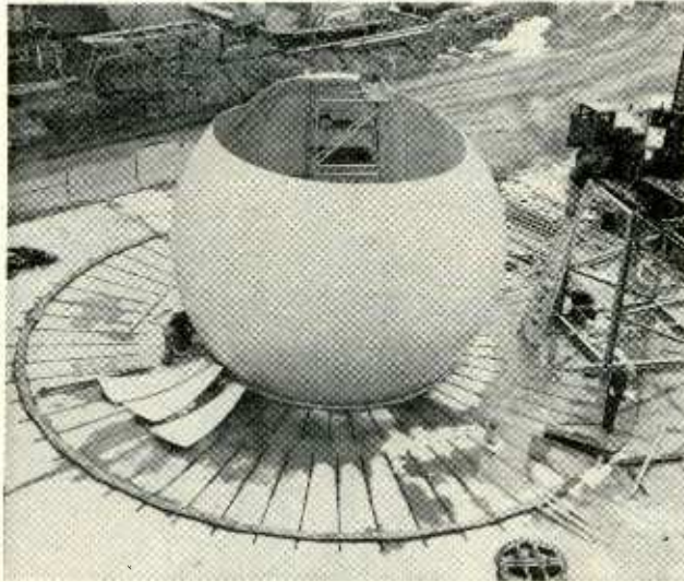
FIG. 1—Preparing the CW-413/FPS(XD-1) radome for structural testing. It is a truncated spherical shell with an equatorial diam of 26½ ft, base diam of 20 ft and wall thickness of ⅛ in. It is composed of 55 panels bolted together
