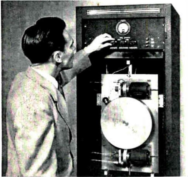
Adjustment of two potentiometers is required to zero system. Because there is little interaction between the two settings, system can be adjusted with one repetition of the two steps
