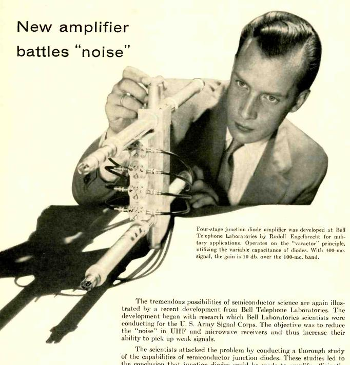
The scientists attacked the problem by conducting a thorough study of the capabilities of semiconductor junction diodes. These studies led to the conclusion that junction diodes could be made to amplify efficiently at UHF and microwave frequencies. This was something that had never been done before. The theory indicated that such an amplifier would be exceptionally free of noise.
