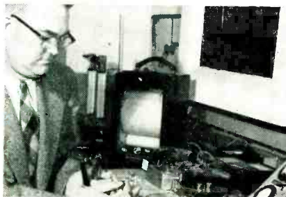
Small transmitter held in hand of J. T. Mengel, NRL scientist, is enclosed in gold-plated aluminum container. Signals from the transmitter will be used to track the unmanned earth satellite of which a model is shown at right. A. V. Astin, National Bureau of Standards discusses Project Vanguard with Capt. B. G. Wade of Office of Naval Research
