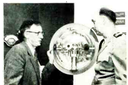
Small transmitter held in hand of J. T. Mengel, NRL scientist, is enclosed in gold-plated aluminum container. Signals from the transmitter will be used to track the unmanned earth satellite of which a model is shown at right. A. V. Astin, National Bureau of Standards discusses Project Vanguard with Capt. B. G. Wade of Office of Naval Research
