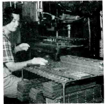
After final treatment, plated strips are cut into individual radio boards on punch press having positioning pins that automatically give accurate registry
