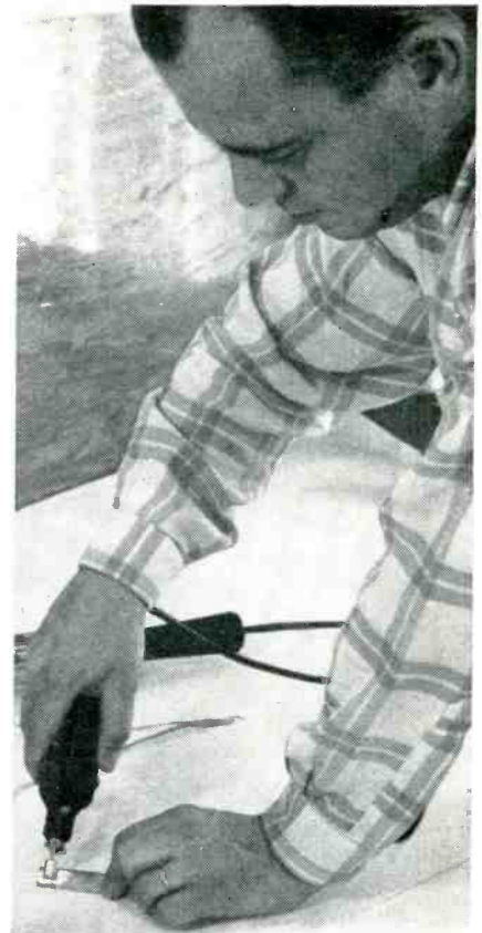
Using loaded wheel to tin piece of stainless steel
