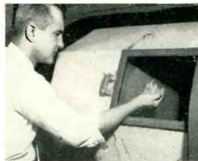
Inspecting parts that have been dried by tumbling in sawdust
