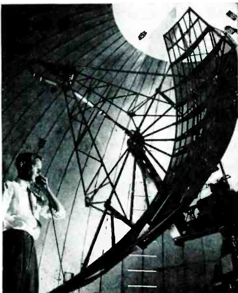
Huge antenna used with new radar height-finder needs a room all its own above the control center in the radome building erected in Arctic climates. Air pressure supports the rubberized glass fabric radome "balloon." Entrance to the radome is through an air lock chamber.
