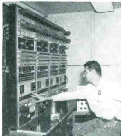
Electronic equipment in new Navy Lab includes 40-channel gamma-ray analyzer
