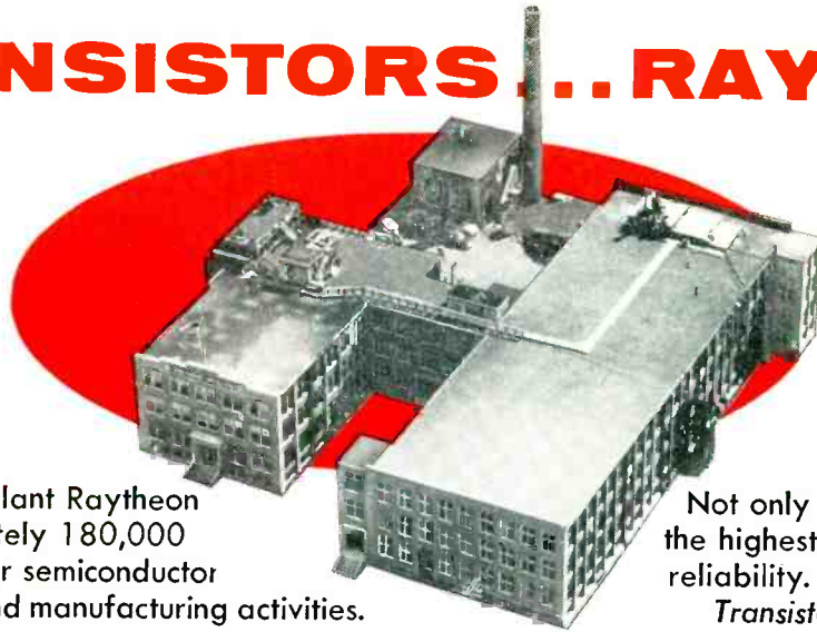
Raytheon's new Semiconductor Division Plant at Newton, Mass.
