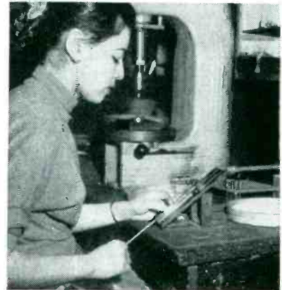
Loading pellets on assembly fixture
