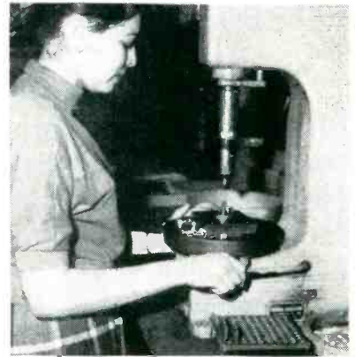
Preparing to operate press after placing loaded housing on bed of press and inserting other lead in die of press
