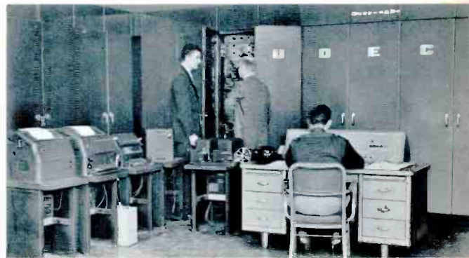
UDEC II, a complex pulse system. The giant Burroughs Unitized Digital Electronic Computer is built entirely from Burroughs Pulse Units connected together with standard cables.
