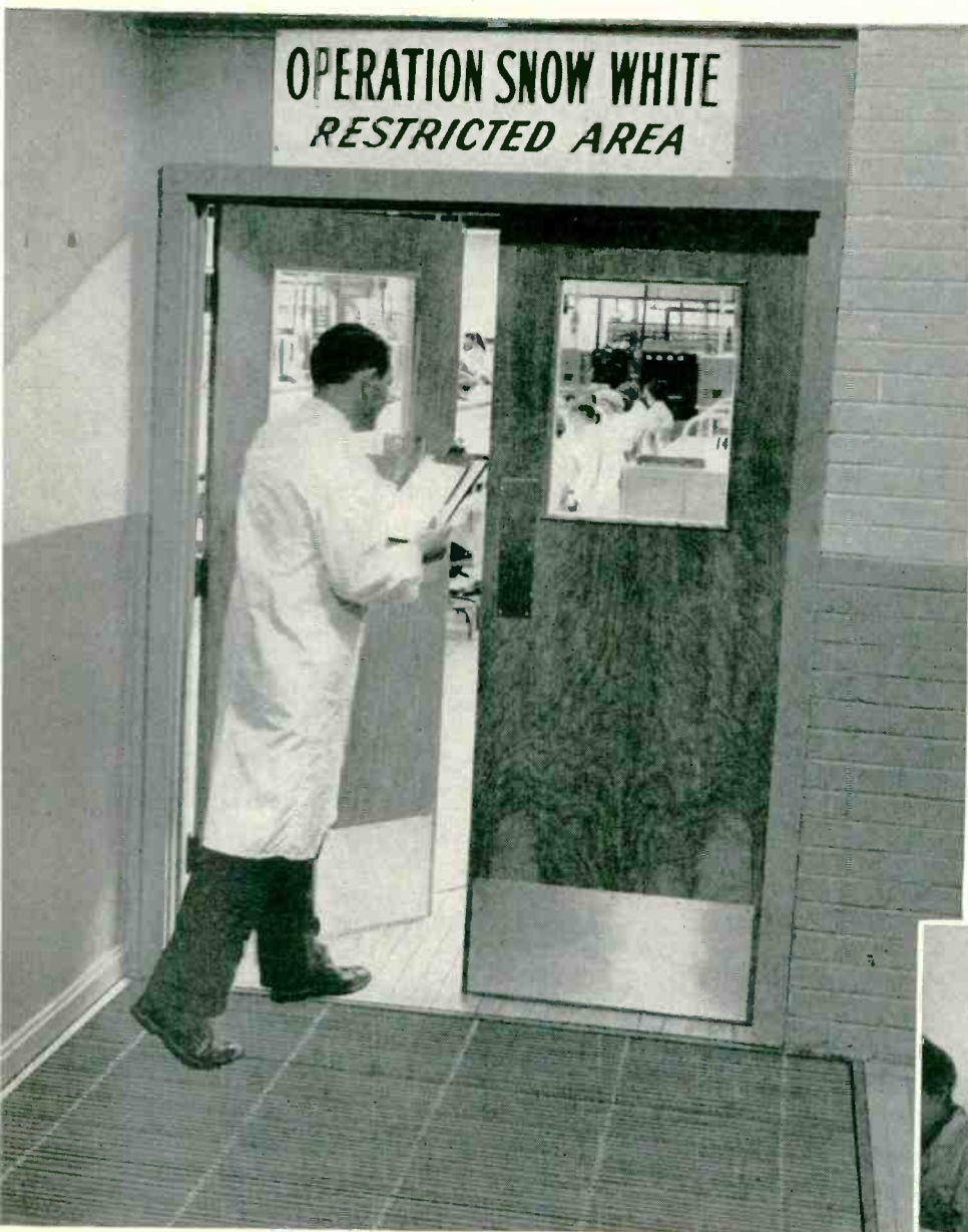
AIR-LOCKS AT ALL DOORS. Employees and other persons entering, pass through air-locks, with a grating underfoot through which powerful suction removes any loose dirt from their shoes. All outer garments, lunches, and personal articles are left outside, in a separate cloak-room. Traffic is closely controlled, and those permitted to enter must wear lint-free clothing. Incoming mail is left in the air-locks, for pick-up and delivery later on by employees who work inside the "Snow White" area.
