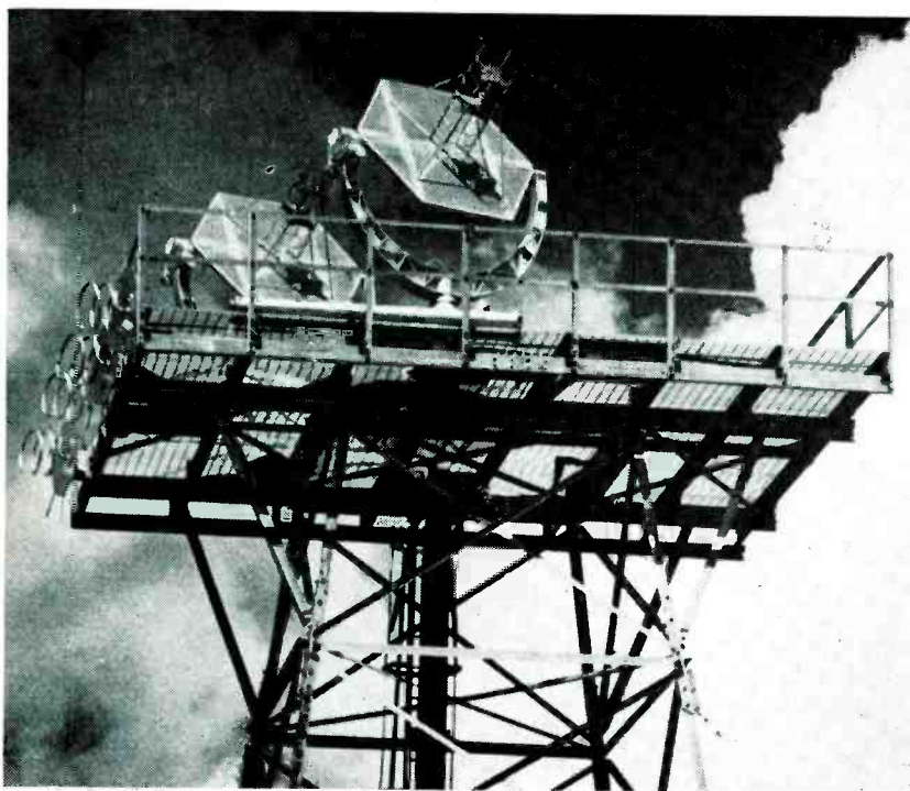
Installation of dual seven-turn remotely tracked helical antennas on 50-ft tower
