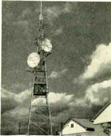
HIGH-GAIN paraboloidal antennas beam microwave signals over 288-mile mountainous path to provide a . . .
