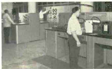
Test benches and control and distribution panels.
