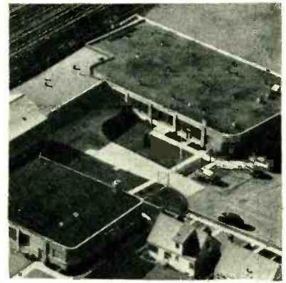
Newly enlarged Volkert plant
