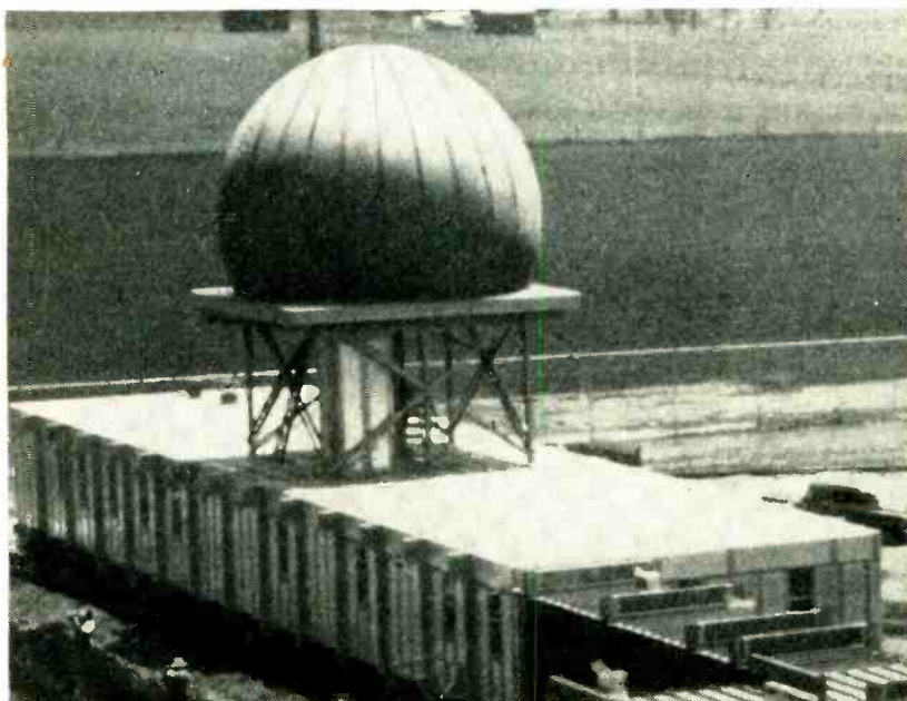
RUBBER DOME protects intricate antennas from weather as . . .
