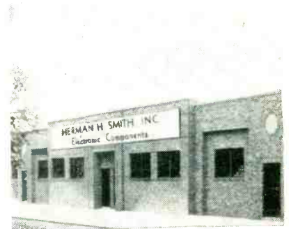
New Smith plant
