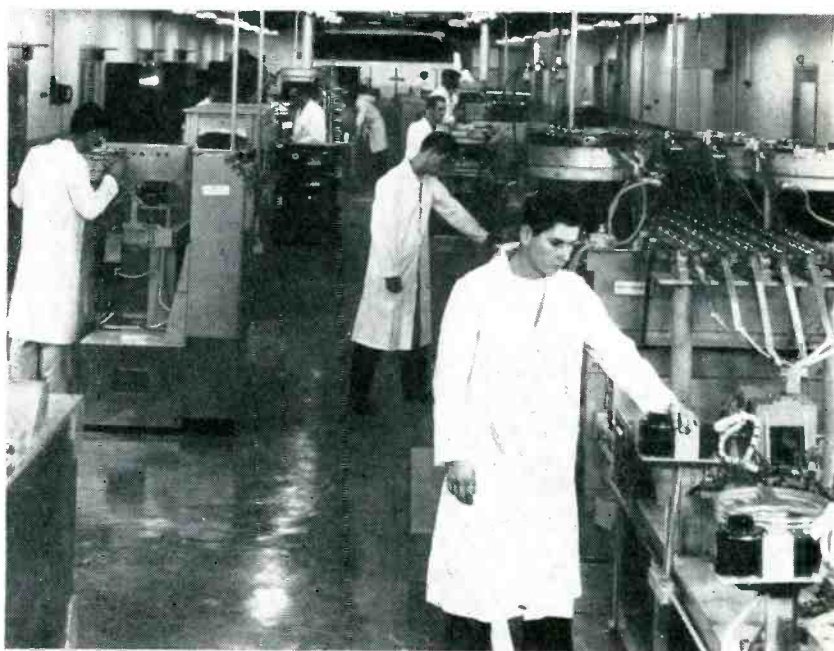
PROJECT TINKERTOY combines printed-circuit techniques and assembly equipment with a system of equipment design so that a . . .
