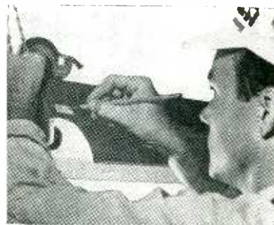
Method of using tape to determine life of fluorescent tubes
