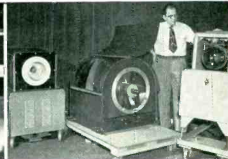
Rauland large-screen projectors using three different optical systems, all of which give theater-size pictures.
