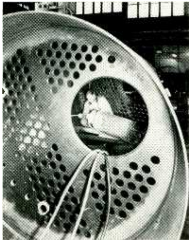
Midget-sized industrial x-ray unit, developed by GE, goes inside boilers to inspect welds. Equipment is part of two-wheel trailer unit that carries power supply and all apparatus
