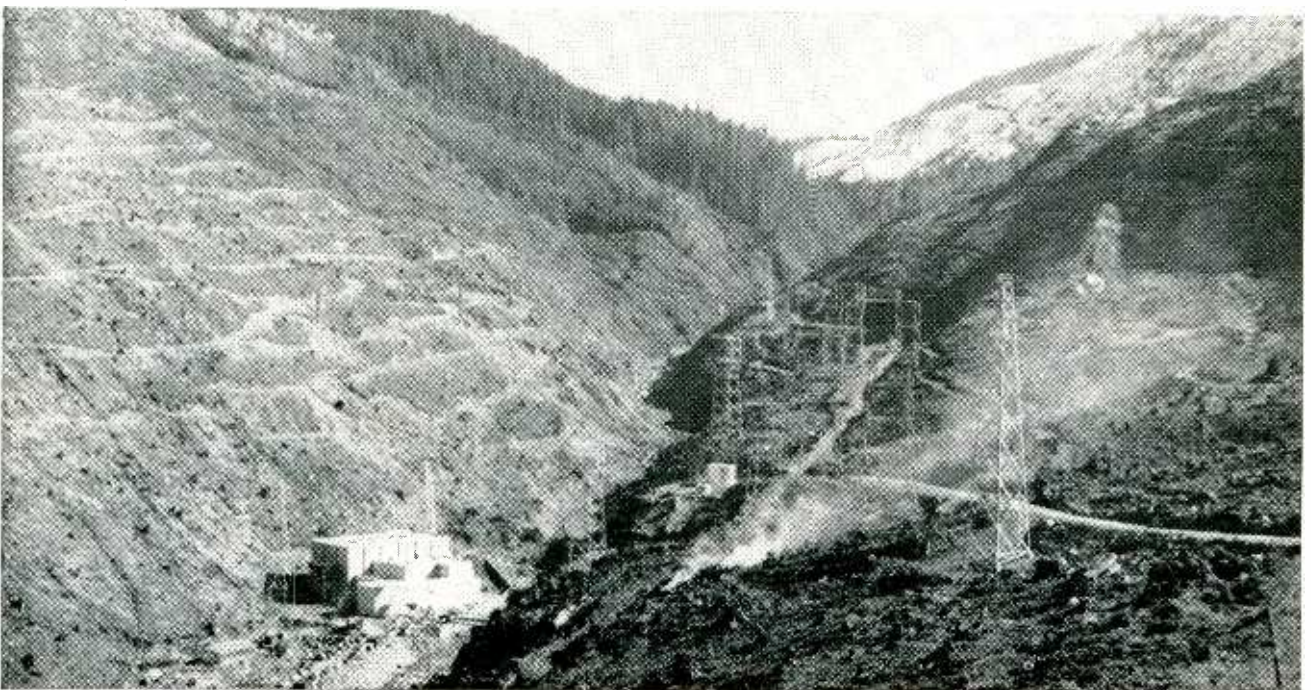
Navy vlf transmitter in Jim Creek Valley will deliver 1,000 kw to catenary antennas suspended between twin 3,000-ft peaks. Open towers (foreground) will carry antenna-feed bus
