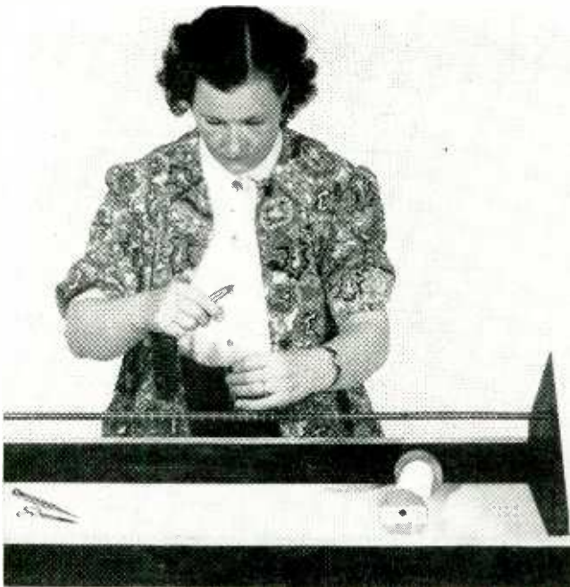
Board used for practicing the forming and soldering of cables
