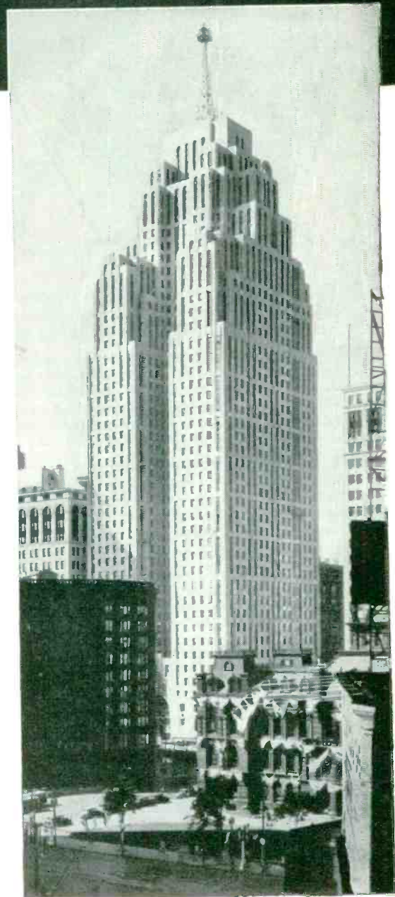
PENOBSCOT BUILDING —Detroit's highest—houses all of WWJ-TV's transmitter equipment. TV antenna tops highest central portion. Here are transmitted programs originating in new studios powered by G-E load centers.
