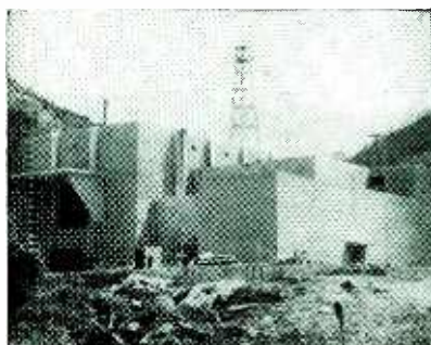
Transmitter building contains dual 500-kw rigs and auxiliary equipment. Structure is copper shielded against intense electromagnetic field
