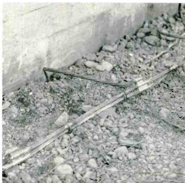
Elaborate ground system is made up of copper conductors. Ground wires take to the air when crossing creek as shown at left. Close-up at right is creek diversion wall and shows one-inch copper conductors brazed to form ground screen
