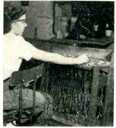
Rolling rack for television receiver line cords. Operator places cords on it after stapling the metal back-cover plate to the female end of the cord
