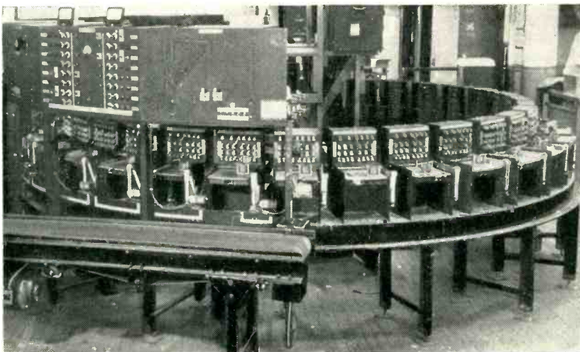
Over-all view of transformer tester. The six different test positions are located above the turntable at the left
