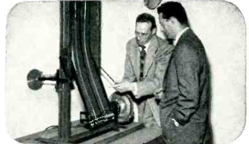
Remember this traffic-stopper at the 1952 IRE Show in Grand Central Palace? It's a torture test. Flexed well over 1,000,000 times, Waveflex flexible Waveguides gave no evidence of failure or loss of physical or electrical properties.
