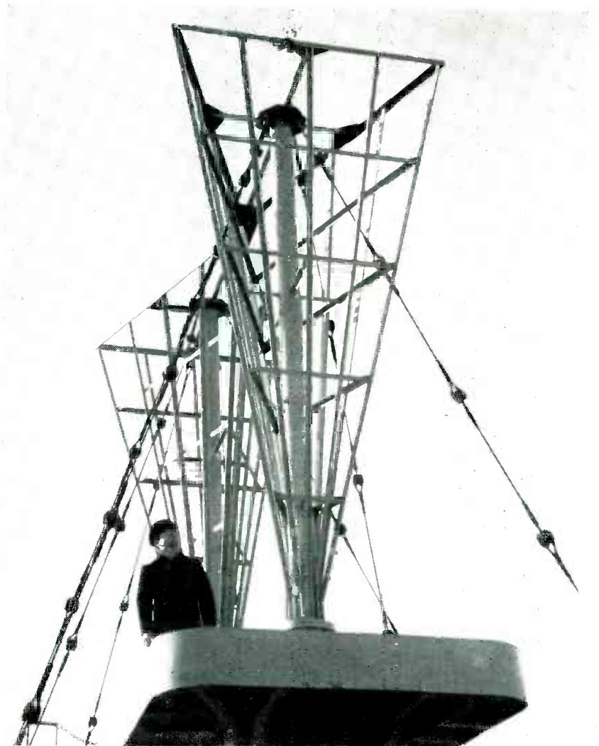
Inverted pyramids are mounted upon special superstructure. One end is grounded and other is mounted upon insulator
