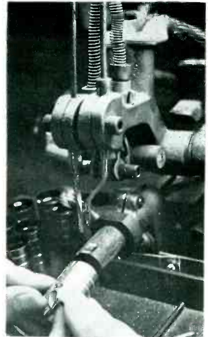
Wood anvil positions getter cup accurately for welding to tube anode
