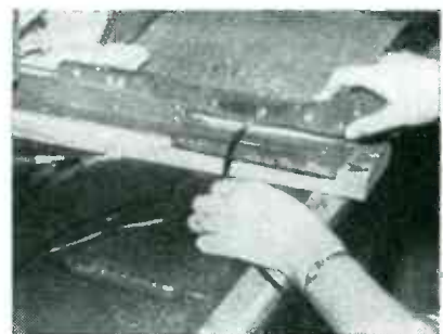
Pulling knife forward to cut shielding braid
