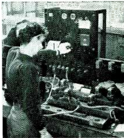
MAGNETIC OVERLOAD RELAYS are tested for tripping time by Anthony J. Bellitto before they are installed on motor control panels.
