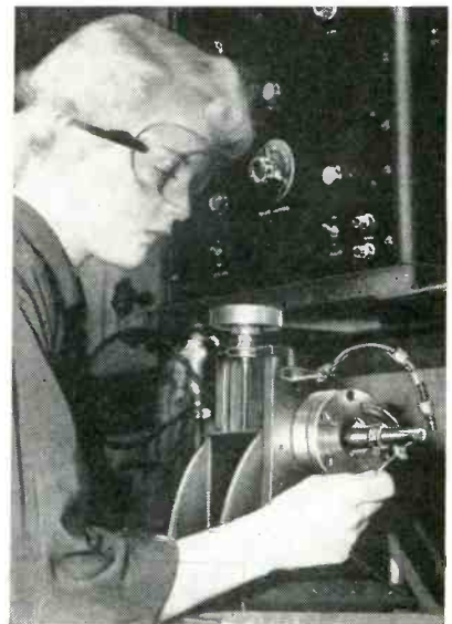
To remove adhering glass, operator inserts rod in hole in end of ultrasonic vibrator
