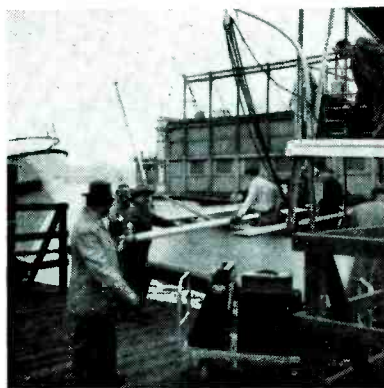
FIG. 2—An attempt to load a generator aboard the ship using an improvised wide gangway. A dock crane actually placed unit aboard, as tide shifted
