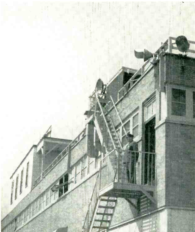
Classified equipment that must necessarily be electrically "in the clear" may be hidden from public view by tarpaper and wood structures
