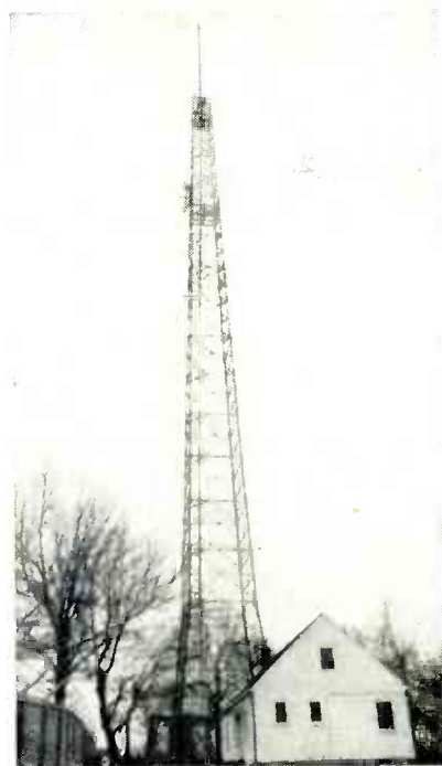
Bridgeport-Stratford uhf station and transmitting tower. Program receiving antenna is at 160-foot level
