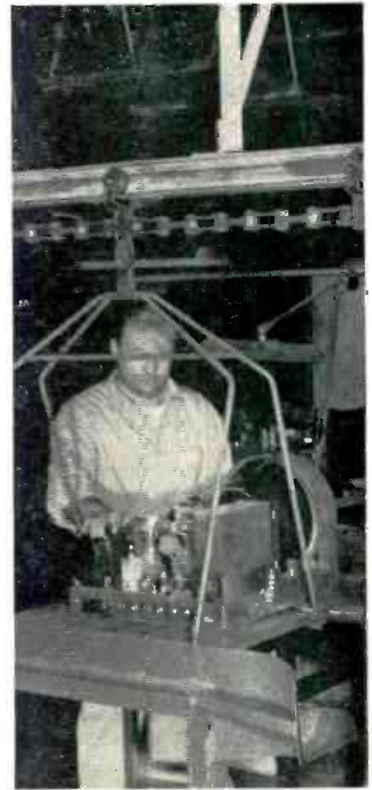
FIG. 5—Overhead chassis conveyor moves between curved guides that hold platform steady as a chassis is slid on or off. This conveyor eliminates lifting and trucking about 40 tons a day
