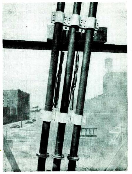
Coaxial cable hangers compensate different coefficients of expansion of steel tower and copper line. Upper clamps cre merely lined with asbestos compound. Lower copper-lined clamps grip coax. Downward thrust is taken by springs. Ground is carried by the copper braid from lower clamp to tower
