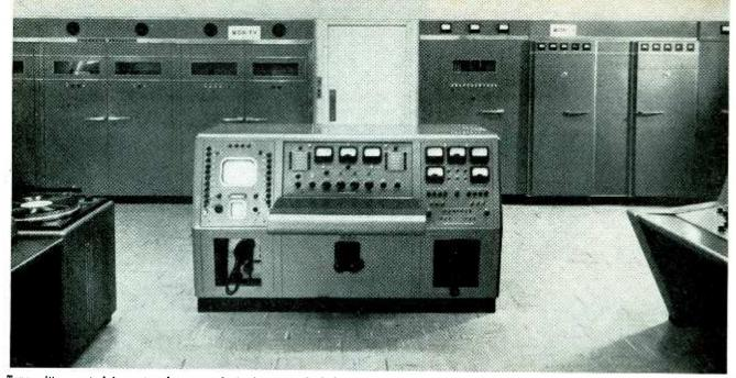
Transmitter control is centered at console in foreground. Television transmitters at left and f-m at right. Turntables and cueing desk just show at left and camera control and mixer desks at right
