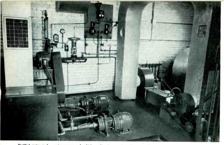
Distilled water cooler, water pumps and cubicle cooling fans in the utility room. Flow control equipment and safety interlocks are mounted on wall at the rear
