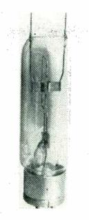
This GE type FH-11 split-anode magnetron was available commercially in 1930 but nobody wanted it
