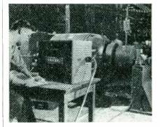
The rotational speed of the turbine is being indicated in the electronic pulse counter. The pulse pickup is mounted on the shaft at the right
