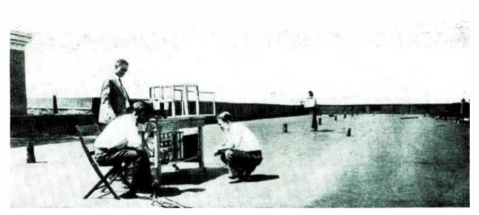
Taken in 1928, this picture shows a laboratory test of the FH-11 oscillating magnetron being used as a voice-modulated microwave transmitter at 400 mc. The art was not ready for such a development, and many years had to pass before a radio
