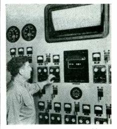
Six glowing discs represent six different flames as viewed by a remotely located camera on the furnace floor
