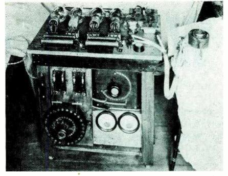
Built and successfully demonstrated by the author in 1919, this high-frequency induction heating unit was 20 years ahead of its time. Commercial acceptance did not come until about 1939 when industry realized its potentialities for surface hardening
