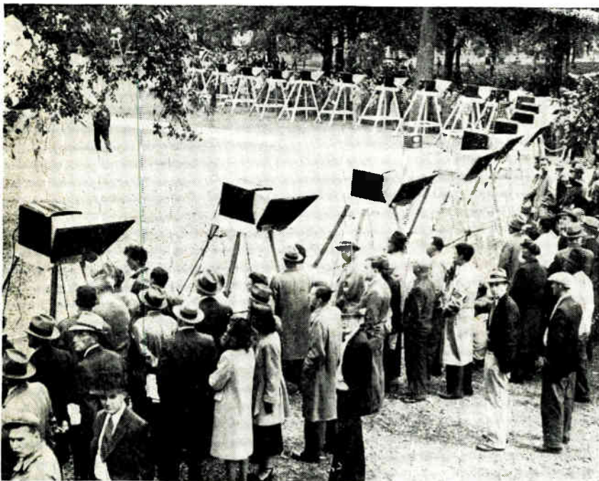
Baseball fans unable to get into the ball park view opening game of World Series over RCA television sets installed by that company on Boston Common. Telecast was from WBZ-TV, Brighton, Mass., with microwave relay and coaxial cable providing feed from the master receiver atop the Ritz Carlton Hotel
