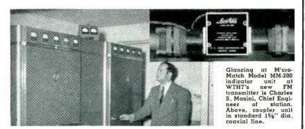
Micro-Match gives you direct, continuous accurate reading in kilowatts. Also gives precise, continuous reading of SWR of antenna system. Thus at a glance you are assured of the proper functioning of the complete RF portion of your transmitter and of your atenna system and transmission line.
