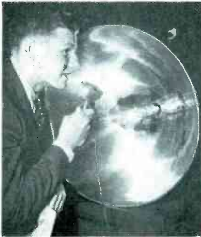
Infrared transmitting tube in reflector, used in Chicago for transmitting a message three-quarters of a mile without resort to wires or radio
