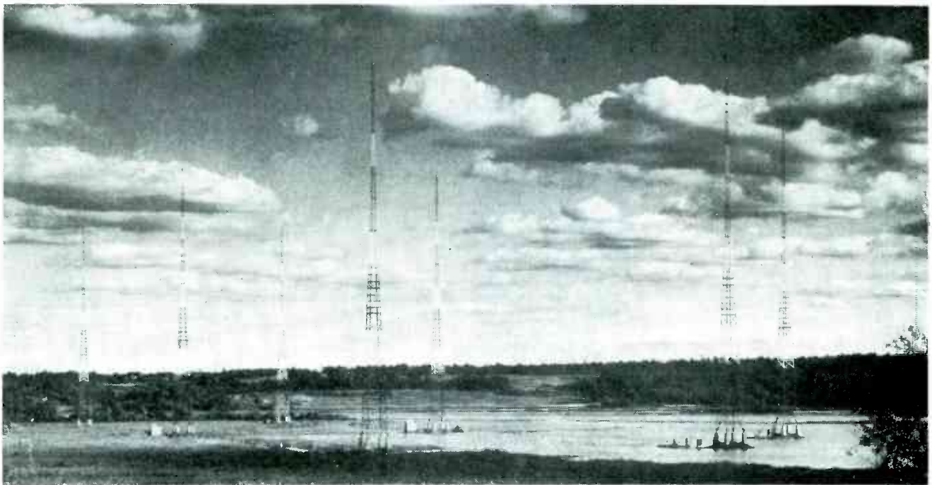
Seven self-supporting base-insulated Blaw-Knox towers, some with wet feet, make up this unusual directional array used by station WREX in Duluth, Minnesota to protect several other stations operating on the same frequency in the a-m broadcasting band. Each tower is 225 feet high. Six are used at night, and the seventh is used with two of the nighttime towers as a three-element array providing daytime coverage over the Iron Range
