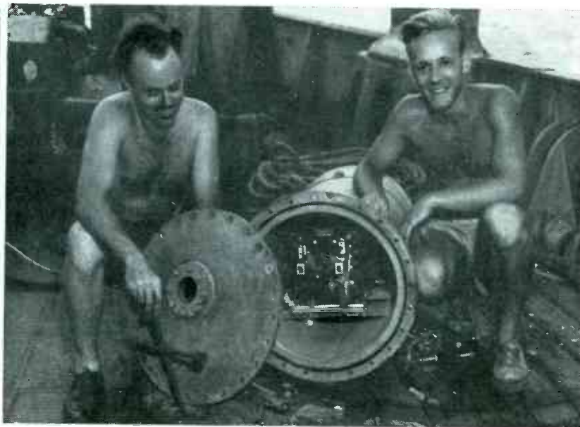
The underwater television camera, inclosed in its steel cylinder. The glass porthole through which it operated may be seen in the cover
