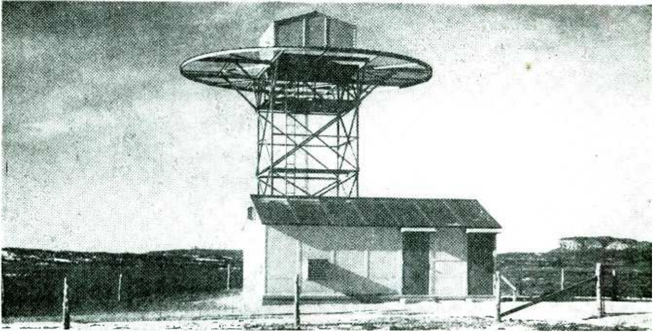
Typical installation of antenna array for vhf omnidirectional radio range. The five loop elements are in the small structure atop the 30-foot-diameter circular counterpoise, and are connected to the transmitter in the building below by means of solid-dielectric cable
