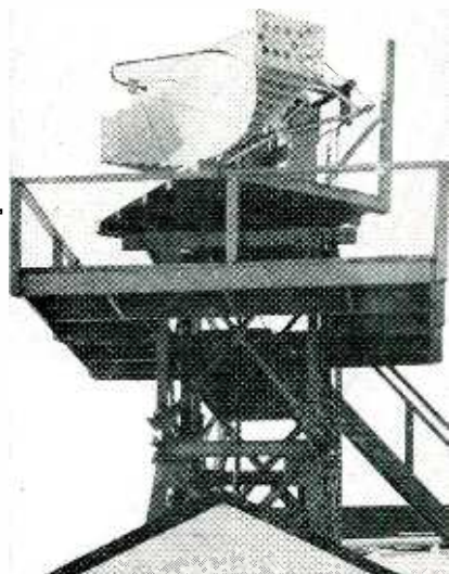
Antenna tower and turntable used in harbor control installation at Halifax, Nova Scotia. The operating room is directly beneath the tower
