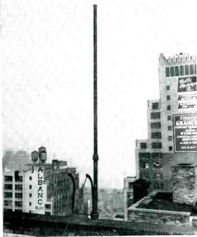
Temporary 152-162 megacycle antenna with a power gain of 3 erected on the Daily Mirror building roof
