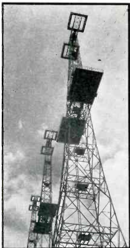
FIG. 1—The radiator of this British CH early warning station is of the mattress-type, supported on 360-foot steel towers. Since 1938 these ponderous stations have guarded the English coast against invading aircraft
