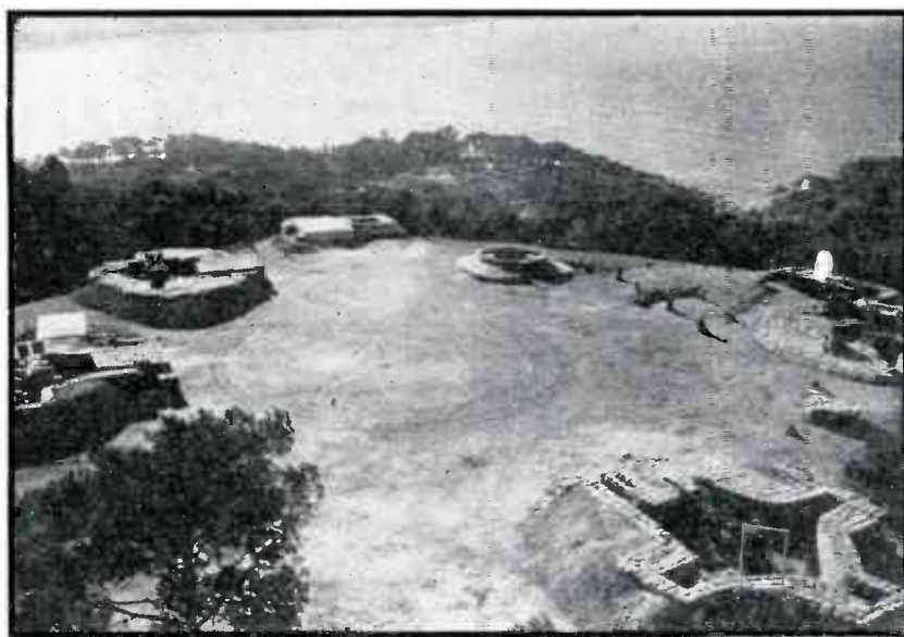
FIG. 11—A 90-mm AA battery protecting the invasion coast in Southern France. The fire-control radar, barely visible at the right (radiator painted out for security reasons), aims the guns automatically with the aid of a computer which introduces the necessary lead. This combination stopped the buzz-bomb attacks on England
