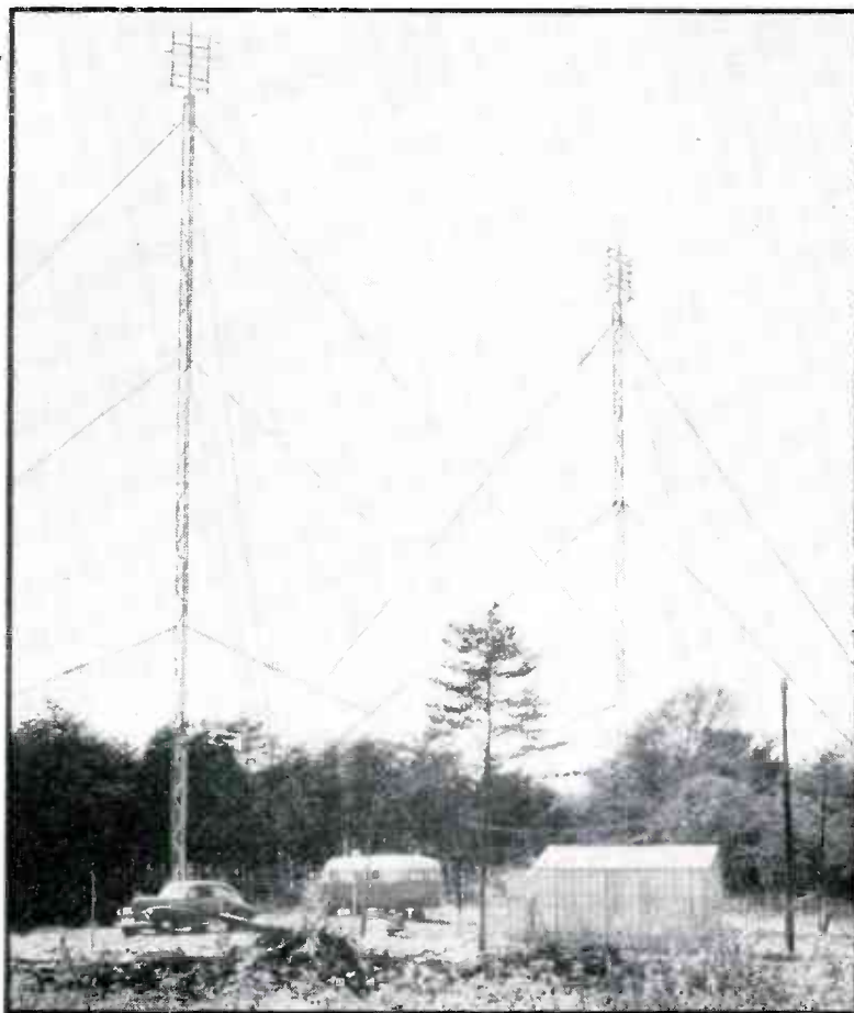
FIG. 3—Relay station at Arlington. The two 100-foot towers supporting receiving and transmitting antennas, the trailer in which equipment is housed, and the small metal building in which tools, spare parts and an emergency gasoline-engine driven generator are kept may be seen
