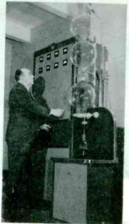
Dr. Brown adjusts the r-f energy being delivered to the penicillin solution during the preliminary evaporation stage in which the dilute solution is concentrated by evaporation at room temperature under reduced pressure
