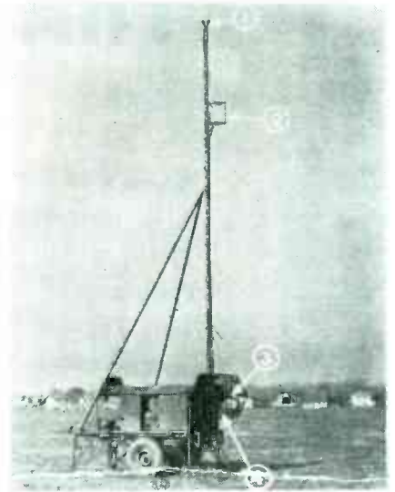
The glide-path transmitter is installed in this trailer. The mast supports an obstruction light (1) and the upper antenna (2). The lower antenna (3) and a screen reflector (4) are mounted at the trailer level
