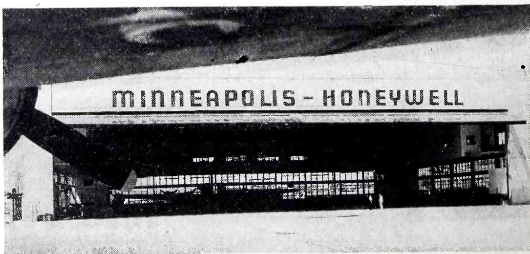
The longest single span truss ever fabricated and erected by the American Bridge Co. went into the construction of this hangar for bombers. Viewed from beneath the wing of a Flying Fortress, the doorway is 34 feet high and 180 feet wide and has no obstructions
