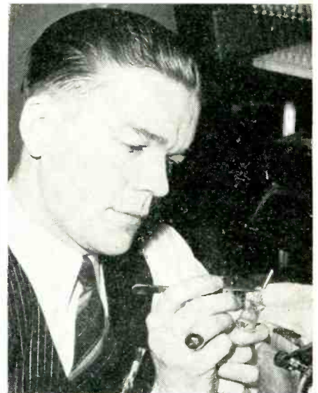
William Hayes examines the spaghetti-supported filament he developed. The spaghetti is made to exact size by a special die
