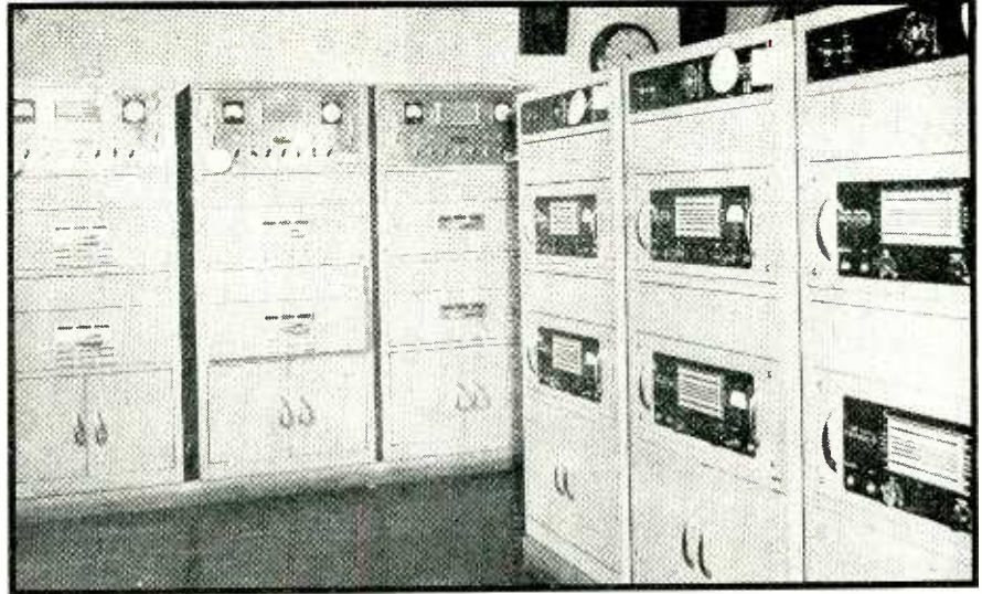
Memovox recorder units, one of which is provided for each program channel on the master control desk, to obtain a reference recording of every program put on the air by OWI. The recorders start up automatically whenever a channel is energized
