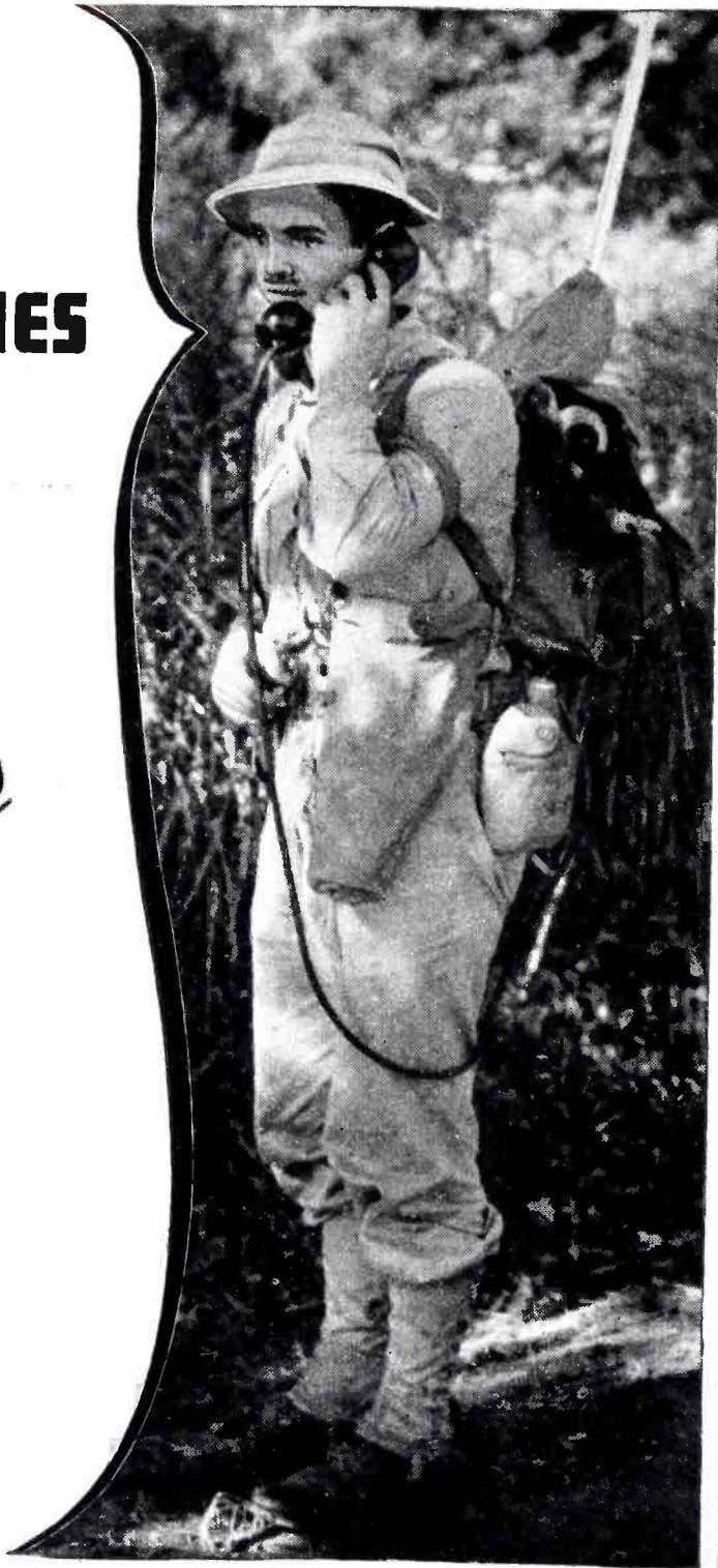
★ U. S. Army Signal Corps Photo. Back-carried Walkie-Talkie two-way voice radio
