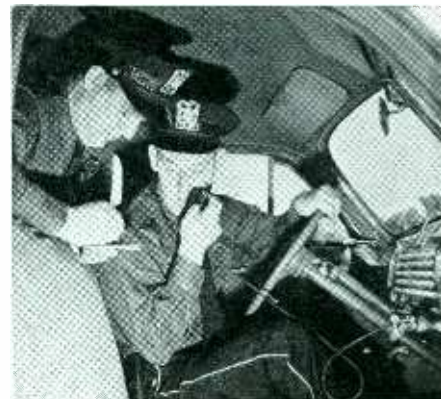
Installation in typical car driven by special Commonwealth Edison anti-sabotage patrolmen
