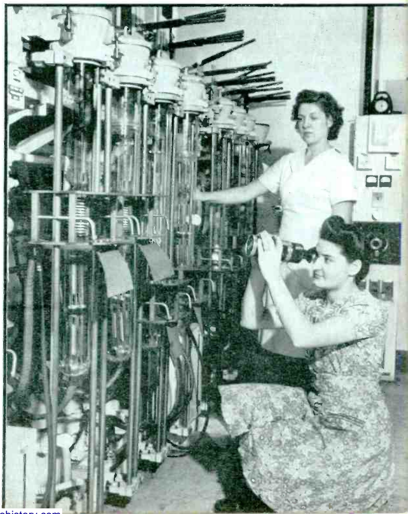
Mary Iatesta and Winnie Ferguson check temperature while exhausting transmitting tubes destined for the armed services
