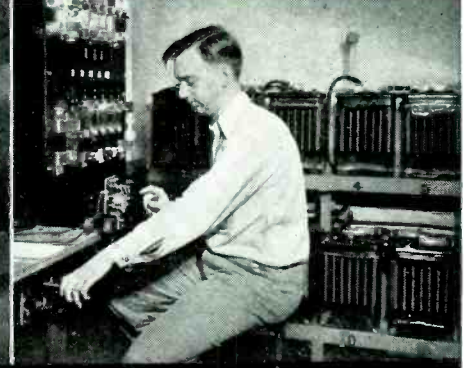
CURRENT . . . Storage batteries delivering any d-c voltage from 2 to 24 volts provide for strenuous load tests. Inrush currents up to 500 amperes and continuous currents up to 250 amperes at 24 volts are obtainable.
