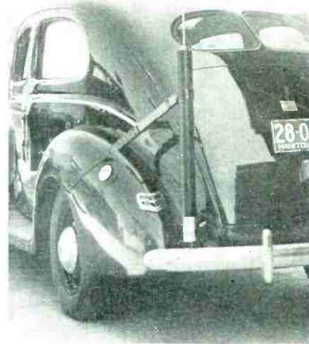
Fig. 3—Solenoid whip antenna attached to rear of patrol car
