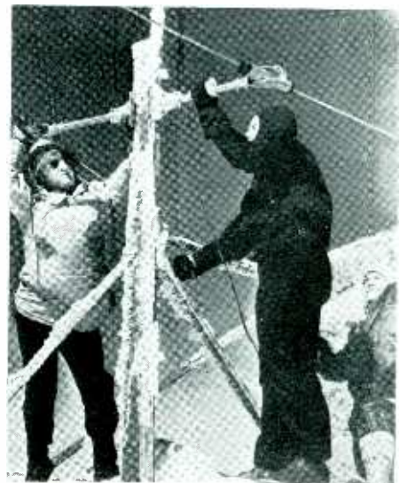
Messrs. Cody, Wiggin, and Corwin erect the television antenna in a 77-mile wind atop the weather observation station
