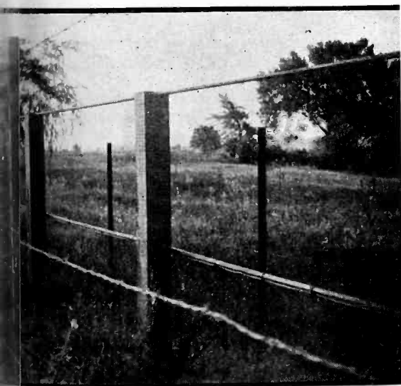
Fig. 12—A 7/8-inch line mounted on slotted posts to allow free movement under expansion or contraction
