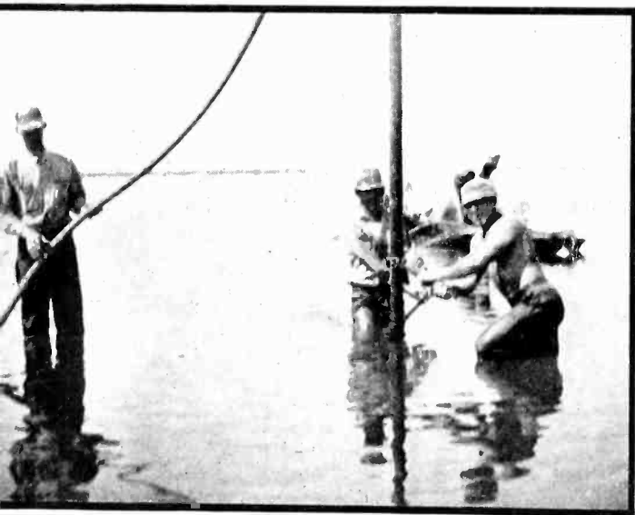
Drilling a hole for dynamite. The landscape is typical of Southern Louisiana at the Gulf
