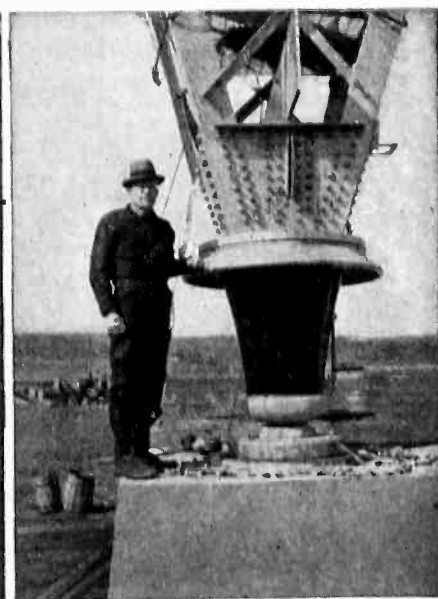
THE TAPERED PORCELAIN insulator at the tower base varies in diameter from 20 inches to 3 feet. It is 4 feet high.
