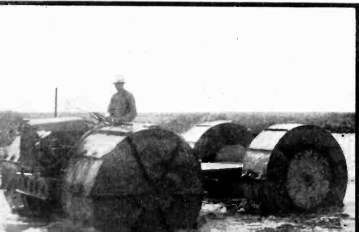
Marsh buggy which is used to transport equipment through marshes and swamps
