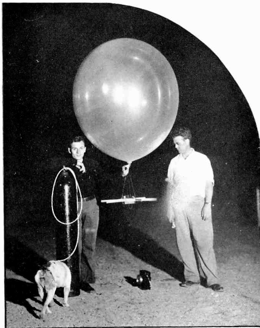
Balloon ascensions at Riverhead determine “angle of arrival” of radio waves
