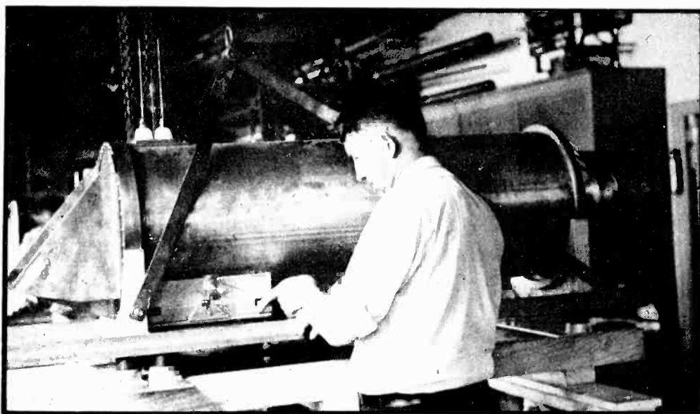
90 megacycle "boiler" transmitter under construction at Rocky Point. At full load the shield gets hot, so air-cooling is used
