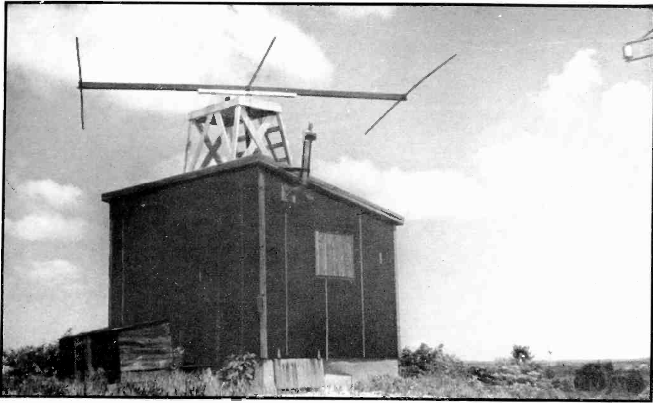
Remotely controlled swivel antenna at Riverhead, used in ultra-high frequency studies
