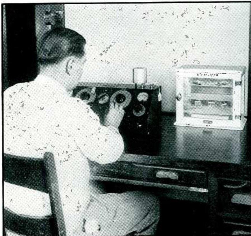
6 A "twisted pair" in position on the Q-meter for measurement
