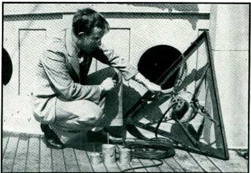
T. J. Hickley of the U. S. Coast and Geodetic survey with the hydrophone unit which detects the arrival of the sound. The three cans in the foreground contain T.N.T. The largest produces an explosion audible for 60 miles
