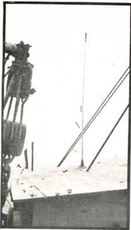
Guyed antenna on Anchor-Derrick barge
