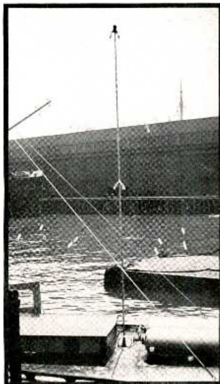
Half-wave rod on 32-foot inspection cruiser "Moreland"
