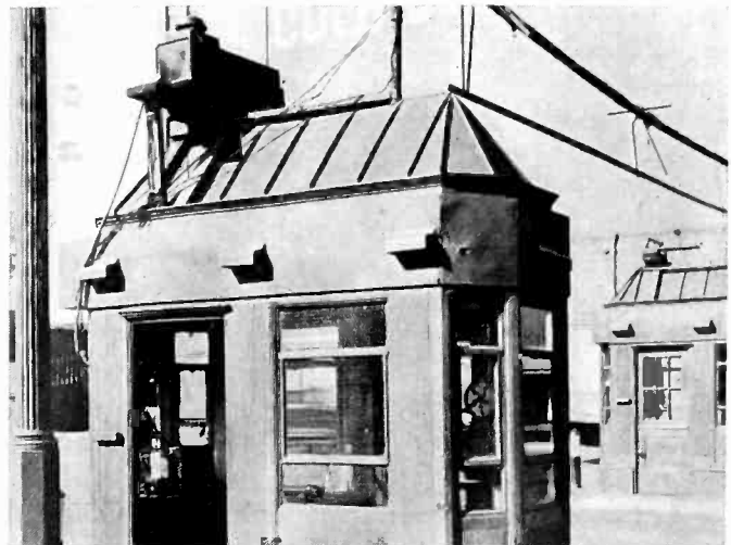
The projector on the nearby toll-house throws a beam into the hooded photonic cell at right. Any intercepting truck starts an alarm ringing
