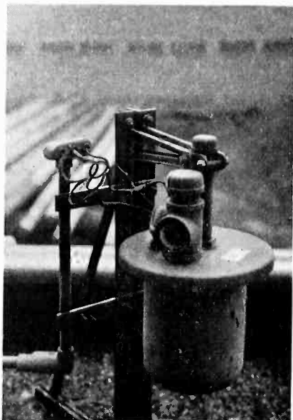
Approximately 50 aviation obstruction lights located on this large storage gas holder in Syracuse, N. Y., are controlled by the G.E. photo-electric tube unit shown
