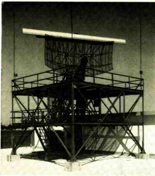
Terminal-radar site showing the cosecant-squared antenna reflector. The horizontal antenna mounted above the radar reflector is the L-band antenna used for radar beacon system.
