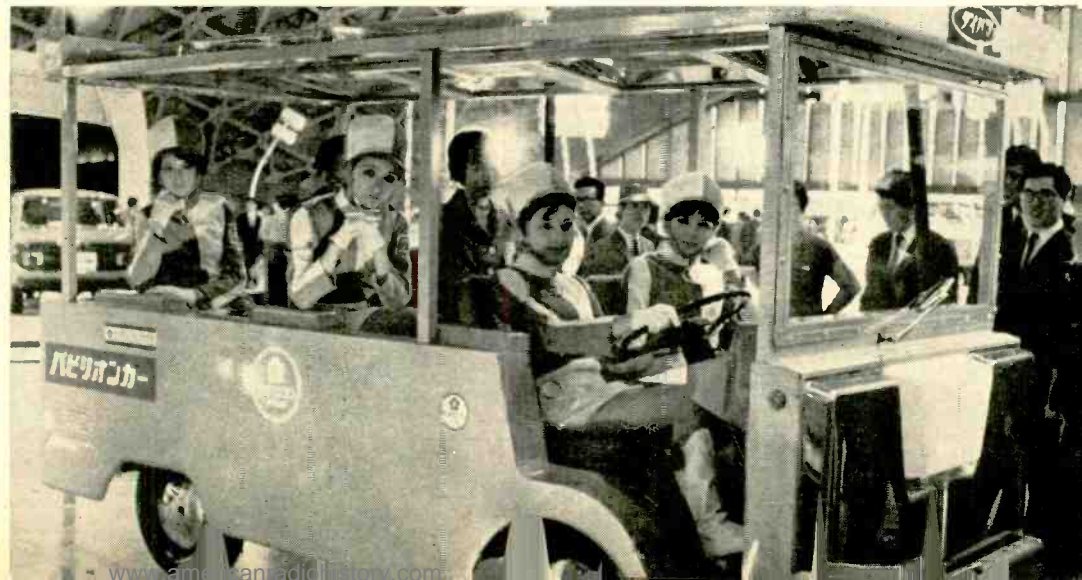
One of three types of battery-powered cars used at Expo '70. All are semi-open and travel at 5 mi/h and will accommodate up to six persons, including the driver. Seventy cars will be used as taxis for fairgoers, 120 cars by distributors, and 10 cars for members of press.
