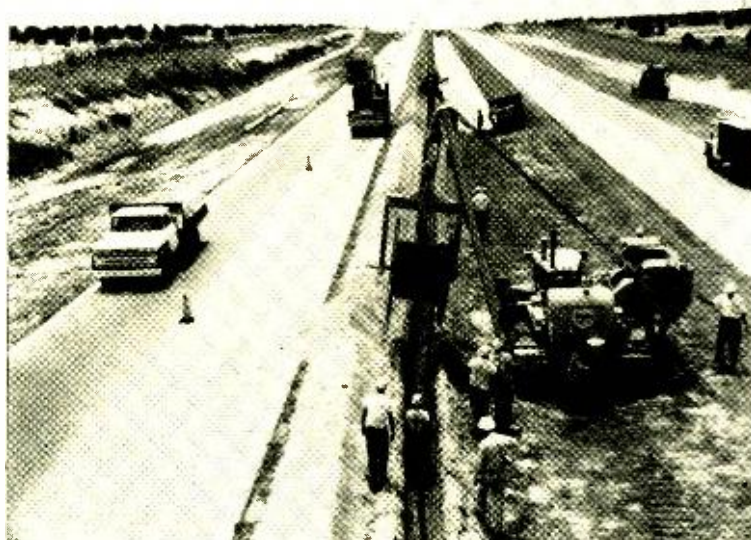
One of eleven bomb-resistant main stations (left) for the L-4 carrier system between Miami and Boston takes shape. The multistory, underground buildings are designed and equipped to operate for several weeks completely sealed off from the outside. Precast concrete manholes are used to house amplifying repeaters. A concrete roof and an 18-inch ground cover will protect the equipment from radiation. (Right) Coaxial cable is being buried to a depth of about 4 feet, where it can withstand overpressures in excess of 150 psi and where most weapon effects are either eliminated or substantially reduced.
