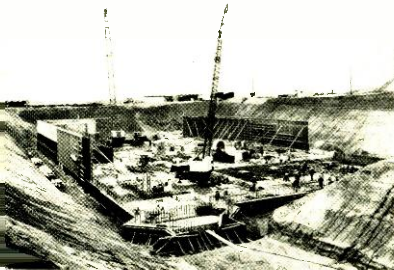
One of eleven bomb-resistant main stations (left) for the L-4 carrier system between Miami and Boston takes shape. The multistory, underground buildings are designed and equipped to operate for several weeks completely sealed off from the outside. Precast concrete manholes are used to house amplifying repeaters. A concrete roof and an 18-inch ground cover will protect the equipment from radiation. (Right) Coaxial cable is being buried to a depth of about 4 feet, where it can withstand overpressures in excess of 150 psi and where most weapon effects are either eliminated or substantially reduced.
